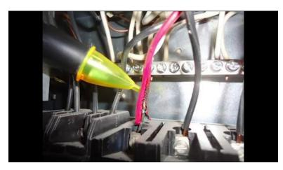
[2m:29s] For example, if you are a wiring, an electrical circuit that can potentially have 15 amps passing through it, you need to make sure that the wire that is being used has an ampacity rating of at least 15 amps.
