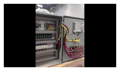
[4m:16s] To assist with this problem, it is important to use wire ties and wire tie anchors which can help in avoiding messy and unorganized wiring situations. The more wire ties that are used, the cleaner the install will typically go. Once again, be consistent in how you use your wire ties. Make sure you use the same size tie and also the same color throughout your install process. Also, make sure to evenly space your wire ties which will give you a
