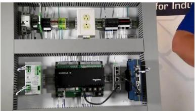
[4m:36s] The next type of terminal block that we've talked about was the ground terminal block. In this particular application, we have one main ground wire coming in and then we have several different components that have grounded on those terminal blocks.
