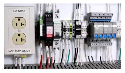
[3m:12s] Single level pass through terminal blocks can also be used anywhere a junction point is required, not just in power distribution.
