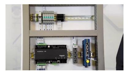
[1m:52s] supplementary protection. The branch circuit protector is located right here. Now, this circuit protector is protecting this entire control panel. So, if I turn this breaker off, it will turn off everything that is located within this panel.
