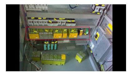
[3m:34s] Some of the common devices that safety relays will be used with are emergency stops, three position devices, safety gates, pressure sensitive mats, contact strips, foot operated switches, and time delay scenarios.
