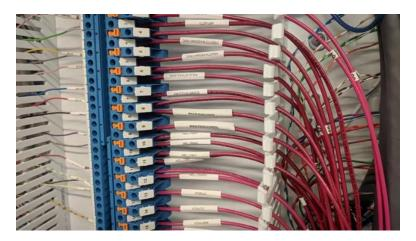
[1m:56s] It is very important that during this step, all of the field wires are labeled clearly and identified clearly so that you or the person landing the field wires understands clearly what wire is associated with a particular signal.
