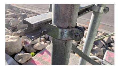
[3m:54s] If you are installing the pole, make sure that the footing is below the frost line if being installed in areas where temperatures can get very cold. It is recommended that the pole being used be made of a very strong rigid material.
