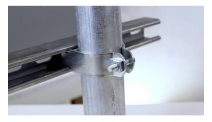
[4m:10s] We typically recommend at least two inch rigid galvanized conduit.
