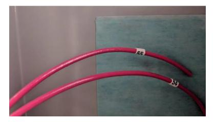
[4m:13s] This allows you the ability to come back at a later point and troubleshoot any problems with much more ease due to the fact that you can more easily identify each wire in the panel as it corresponds to that same wire at the device or instrument termination points.
