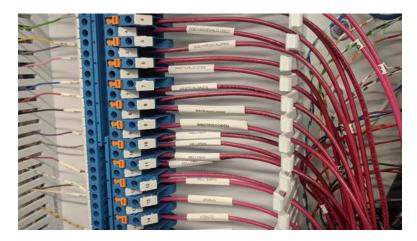
[2m:3s] It is critical to make sure that each wire is labeled with a unique number or letter so that it does not get confused with other wires on the job site.
