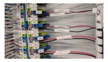
[1m:46s] With the amount of wires that can be pulled on a single job site, having wires labeled improperly or not at all can make this work almost impossible and will greatly increase the amount of time and stress you put on yourself and those working around you.
