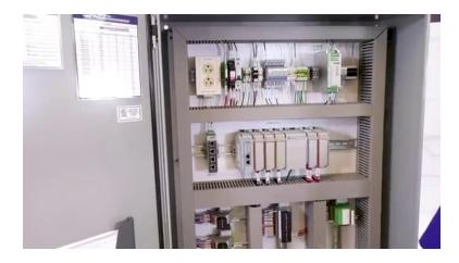
[1m:19s] Voltage should also be checked throughout the panel to make sure the components are seeing the proper amount of voltage where and when it is expected. This is also a good time to check to ensure that any communications equipment is functioning properly as well. This would include the network switch and radio.
