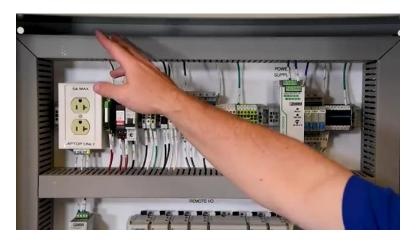
[1m:6s] Power typically comes in at the top of the enclosure, so we typically like to locate our main circuit breaker at the top of the enclosure either on the left side or the right side. We typically see these mounted on the left side.
