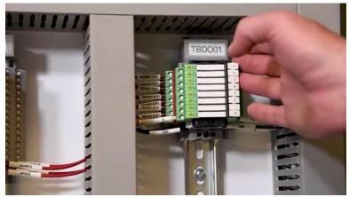
[4m:40s] All of the components within the panel including the wire ducting and din rail, our main to what we call the back plate. The back plate is separate from the actual electrical enclosure itself, and what the back plate allows us to do is fabricate, build, and wire this panel separate from the enclosure.
