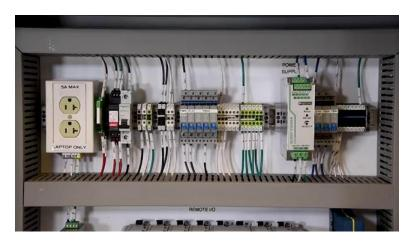
[1m:42s] This is simply where we bring AC power from our main breaker over to this bank of circuit breakers. We have one wire coming in and it connects all the circuit breakers with this jumper bar here. We then send power, AC power in this case, to the components that require AC power within this panel. One component that requires AC power
