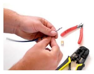
[2m:0s] Once I have that PullString cut I'm going to start separating the individual pairs of wire within the network cable.
