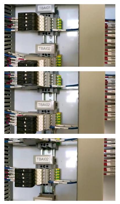
[3m:9s] typically within the control panel where the conductors are being terminated and not at the field side of the device.
