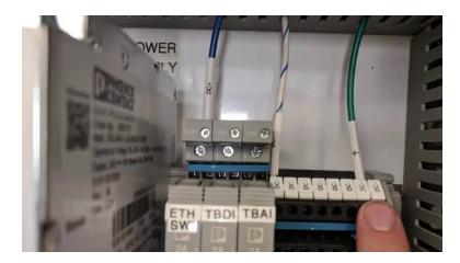
[2m:1s] This location is where the main utility power will enter the panel and is also where the main ground conductor will be brought into the panel as well.
