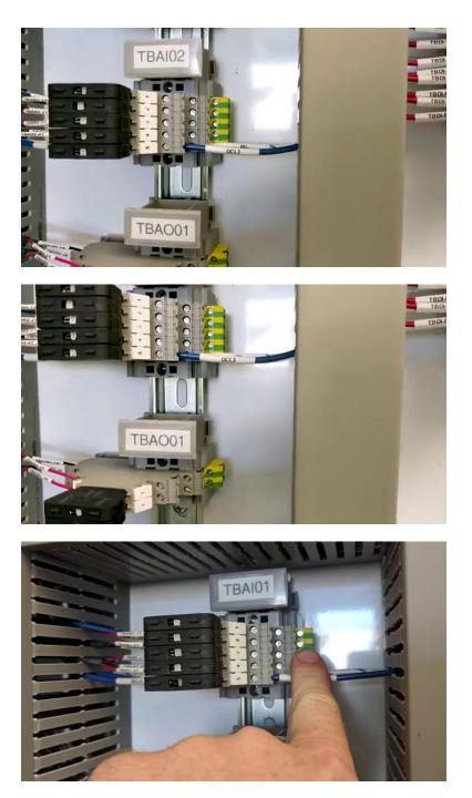
[3m:17s] If both ends of the shielding are terminated, it can create issues with the signals as well as create potential ground loops.
