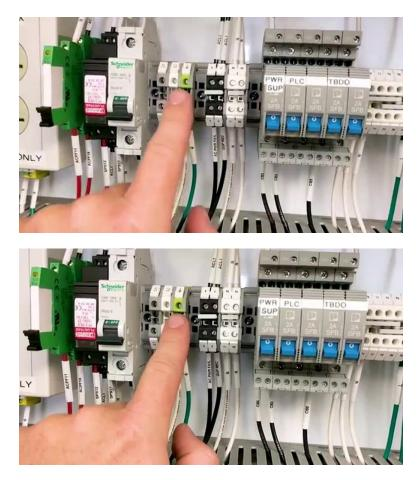
[4m:9s] Lastly, when an industrial control panel is being installed in an outdoor location or anywhere that might be exposed to the elements. It is critical to install a ground rod and ensure that that enclosure is tied to that ground rod.
