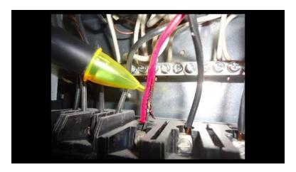
[3m:33s] It may be best to disconnect the power before checking for loose connections on the circuit you are working with. With that said, this is a very common problem and should be checked when you are trying to determine why your circuit is failing. Lastly, a great tip to follow is to always check for short circuits, especially in situations where you are seeing intermittent power surges that are blowing fuses or tripping circuit breakers. Depending on the complexity of your system,
