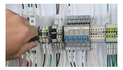
[2m:58s] But, it is not uncommon to find that the source of electrical trouble is many times a loose wire connection. If you are having intermittent continuity issues, this might be a hint to determine if this is your problem. A good way to check for loose connections is to pull test the wire that you suspect might be causing the problem.
