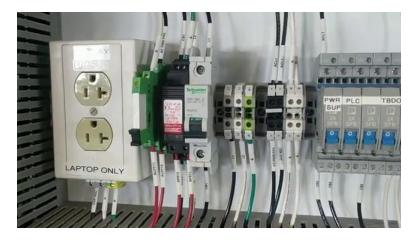
[1m:34s] This can be a device such as a circuit breaker, a fuse, disconnects, and relays. Make sure they are functioning properly. Ensure that the proper voltage is being supplied.
