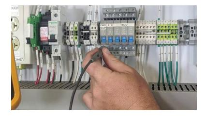
[2m:6s] when electrical circuits aren't working, verify a proper return path. Whether working with AC or DC power, it is essential that a return path is present, such as a neutral wire in low voltage AC circuits, or DC negative or ground wire in DC circuits. Without this return path, the circuit will not function as intended.
