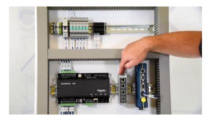
[5m:41s] It also provides better protection for that specific device because the protection being used is sized for only that device. Using supplementary protection in this way does require more time, money, and space in the panel, but is by far the best way to distribute power to the various devices throughout the enclosure.
