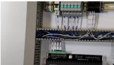
[3m:7s] It is important to always plan your wire ducting to have extra room available once all wires have been run through it, including field wires.
