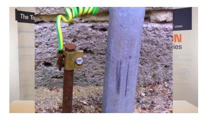
[1m:48s] The size of the ground wire should pertain directly to the short circuit current ratings of the system and the overcurrent protection devices in use. So, make sure to select the properly sized grounding wire for your system.
